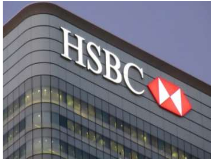
Project: HSBC System: Parking & Access Control
