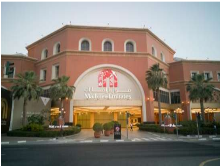
Project: Mall of the Emirates System: Structured Cabling of (CCTV, ACS, Intercom, BMS & AV)
