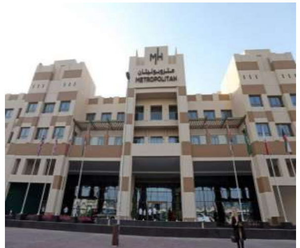
Project: Metropolitan Hotel System: Structured Cabling of (CCTV & Access Control)
