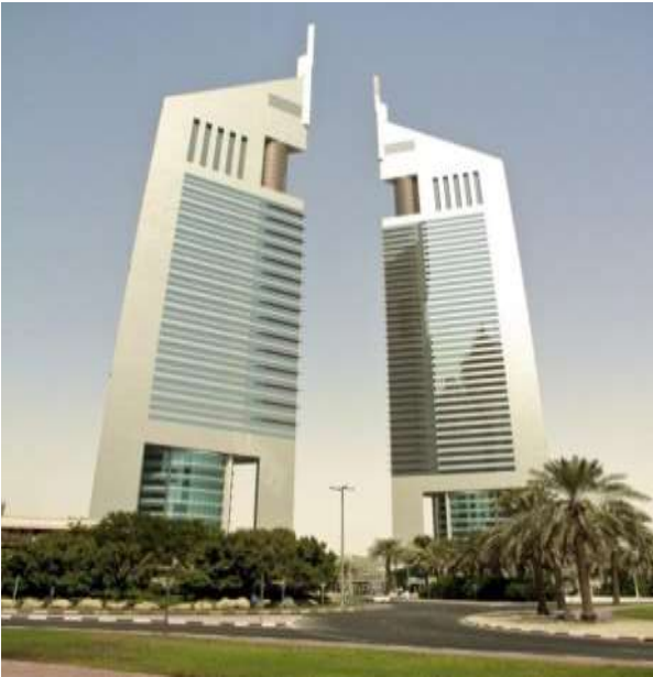
Project: Emirates Tower Systems: Structured Cabling Installation: Worked as a Subcontractor
